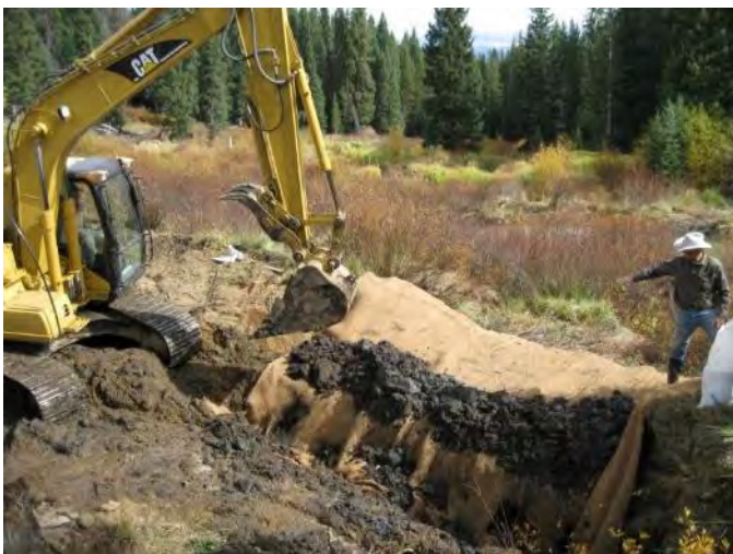
Figure 67: Breached dams were “plugged” with soil lifts wrapped in coir fabric and sod interwoven with live willow stems
