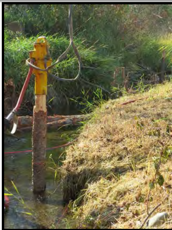
Figure 25: Hydraulic post pounder options. Options include, clockwise, starting from upper left: (a) a hand-held pounder attached to hydraulic power pack, (b) a post pounder attached to bulldozers, (c) a handheld pneumatic post pounder attached to an excavator and (d) a modified excavator with a vibrating pad. Options (a) and (b) take approximately 5 to 10 minutes per post, depending on substrate, and it can be difficult to get to the desired depth. Option (d) takes less than 1 minute per post and can drive posts as deep as needed. All pounders have a metal cylindrical cap that holds the post in place while pounding. Each option has pros and cons to consider, including cost, maximum depth the posts can be pounded, substrate type, operator strength and expertise, and the amount of likely riparian and instream disturbance. Photo credits: (a) Nick Weber, Ecological Research, (b) Mark Cookson, USFWS, (c) Peter Thamer, Siskiyou County Resource Conservation District, and (d) Julie Ashmore, Okanogan Highlands Alliance.
