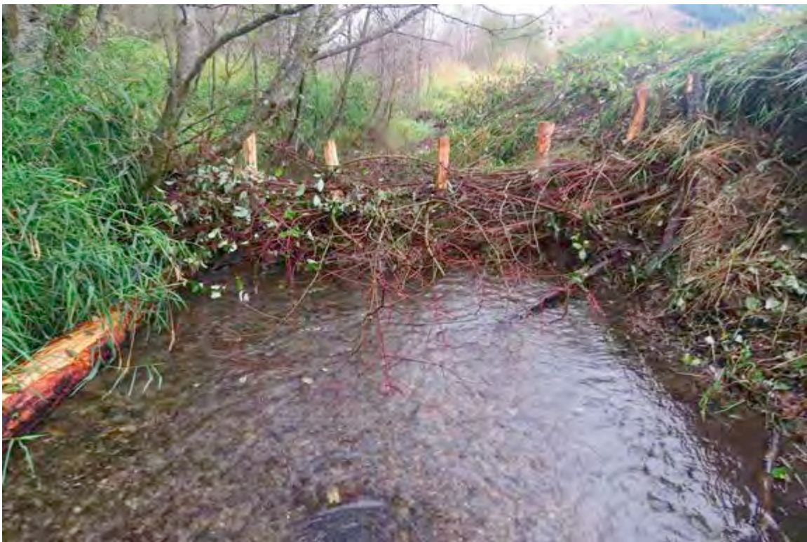
Figure 80: Pilings woven with live red oyster dogwood, some of which was planted directly into the exposed bank to facilitate resprouting
